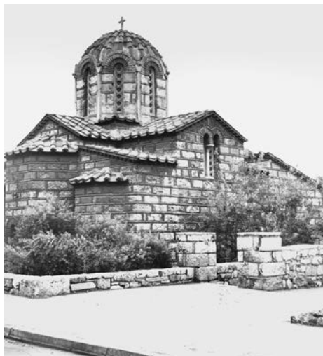
Figure 99 Hagioi Asomatoi near the 'Theseion'. View from the northeast.
